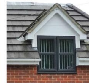
Gable dormer with painted timber casement window.
