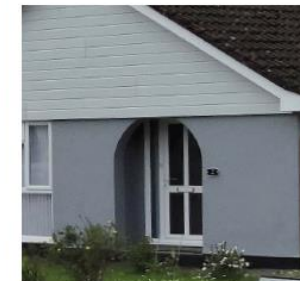
Arched inset front doorway.
