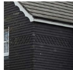
Continuous pattern in weatherboards and decorative fascias.
