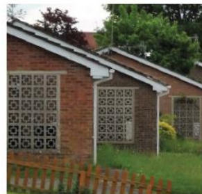
Decorative concrete panes in brick porch wall.
