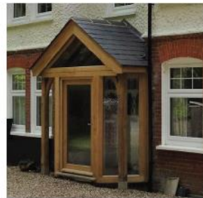
Gable portico with timber frame and glazing.
