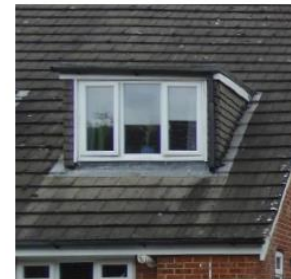
Flat roof dormer with casement windows.
