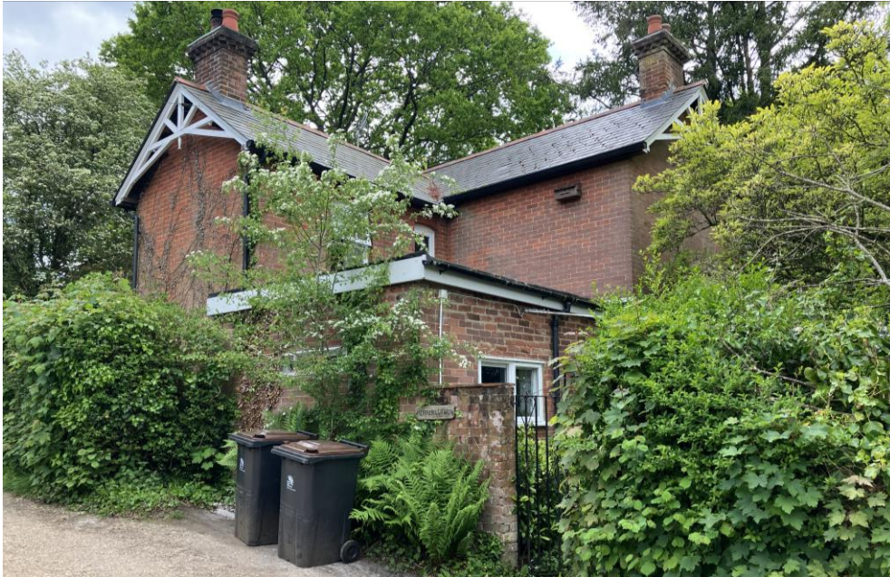
Figure 13. Decorative gable end, ridge tiles and chimneys
